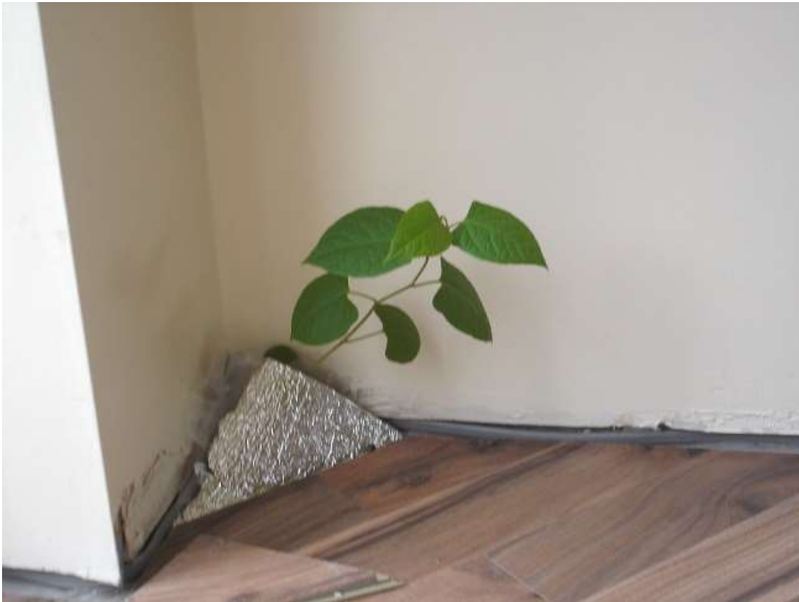
Photograph A.2 Japanese Knotweed having gained internal access to a private dwelling in Co. Cork (Source: O' Donovan Agri-Environmental Services)
